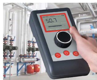
Find compressed air leaks using ultrasound
