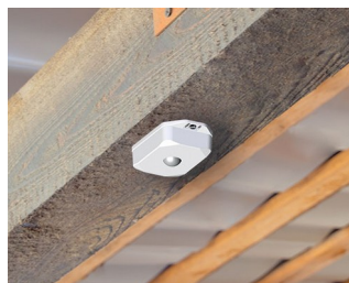
Motion detector with sensor for automatic control
